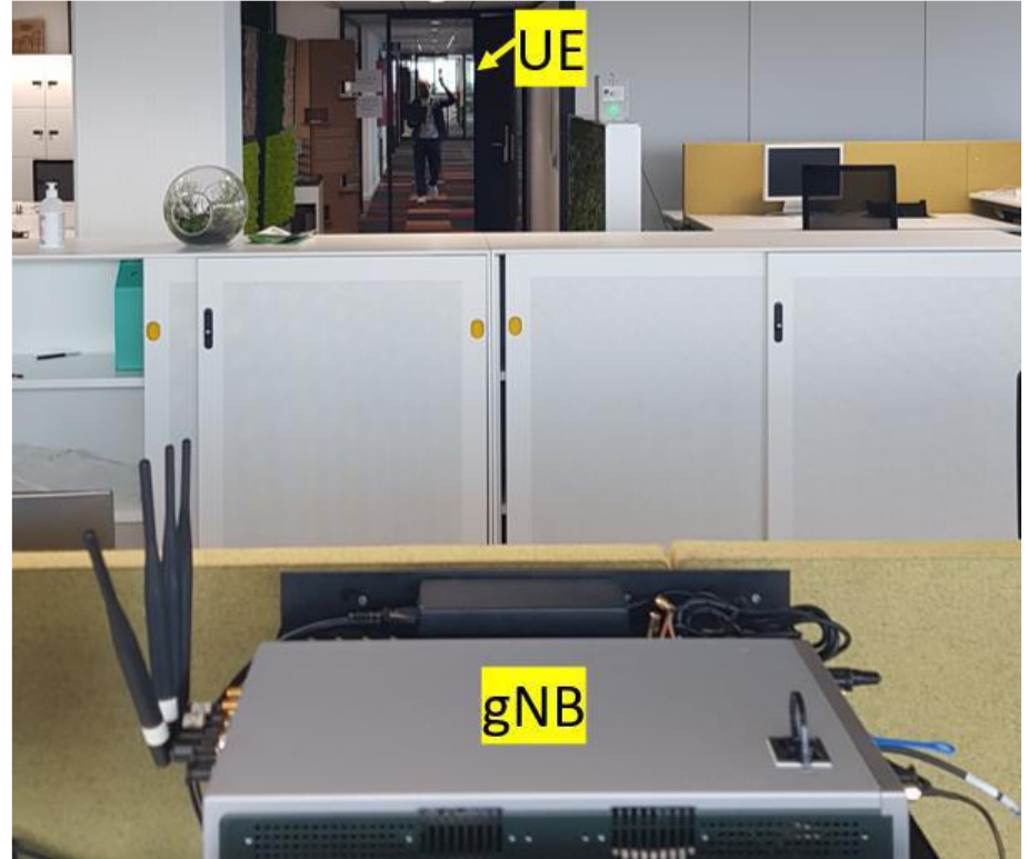
5G NR SA indoor testing using MIMO 2x2, 60 MHz bandwidth and reaching DL 240 Mbps.
